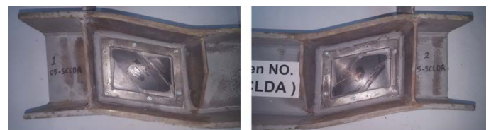
Figure (16): CFRP Separation and slippage in both shear zones for beam (05-SCLDA)
